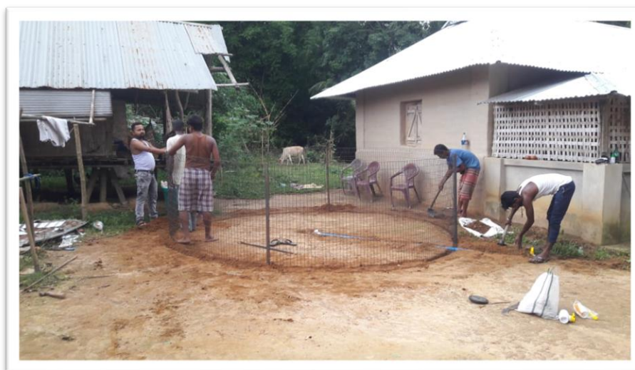
Construction of Tarpaulin based circular Tank
